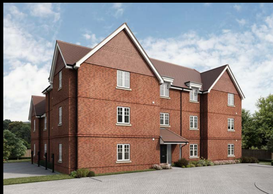
Orchid Apartments 1 & 2 bedroom apartments
